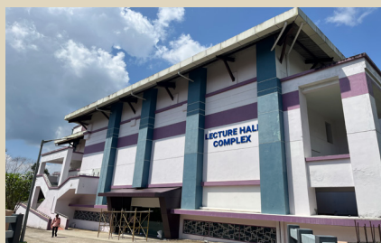
Lecture Hall Complex
